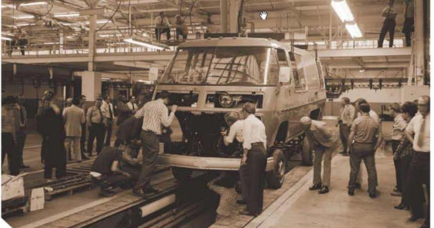
While the racy, flared fenders of the initial scale model were shaved from the production version, the GMC Motorhome adhered to its original and innovative concept. The completely redesigned chassis and powertrain resulted in home-size interior space with car-like handling. The aluminum and fiberglass body was assembled in the same manner as a jumbo jet.
